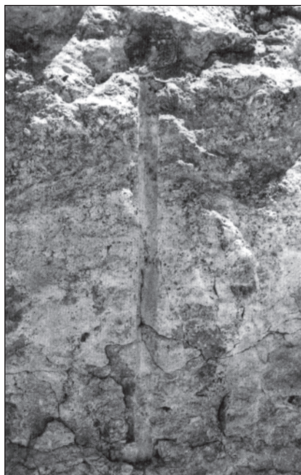
Fig. 10: A running drill mark
