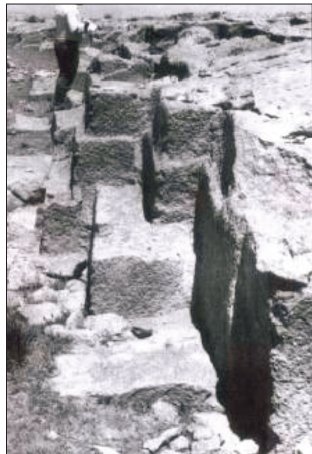
Fig. 7: Vertical quarrying at Al-Istiqlal Street quarry showing the general geology of the area.
