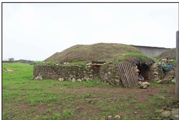
Fig. 4: The cattle enclosure is built of stones, wood and covered by heavy grass.
