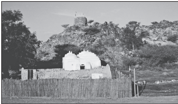
Fig. 2: Bidyah mosque & Tower I, prior to restoration.
