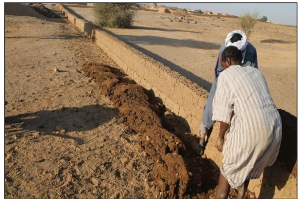
Fig. 15b: Building of the mud wall in process.
