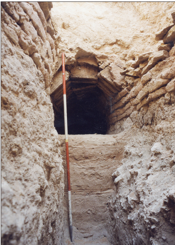
Fig. 3b: Section of Falaj 1 looking northwest. Photo: al-Tikriti.
